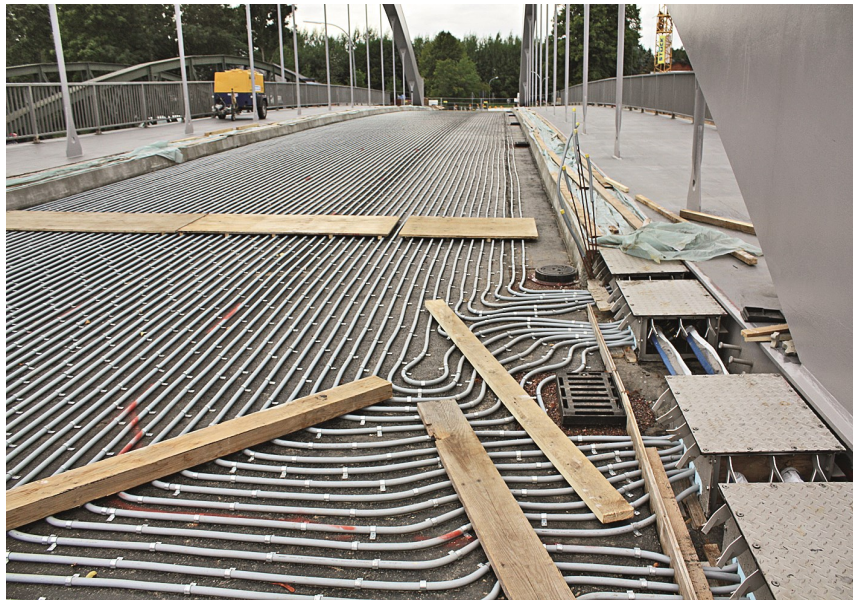
Heating coil embedded in geo-thermally heated bridge, Berkenthin, Germany
