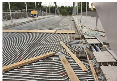
Heating coil embedded in geo-thermally heated bridge Berkenthin, Germany Picture: H.S.W. Ingenieurbüro Rostock
