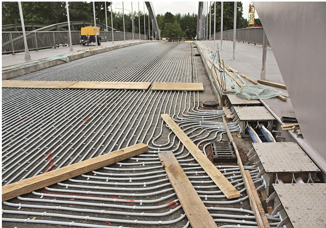
Heating coil embedded in geo-thermally heated bridge,
